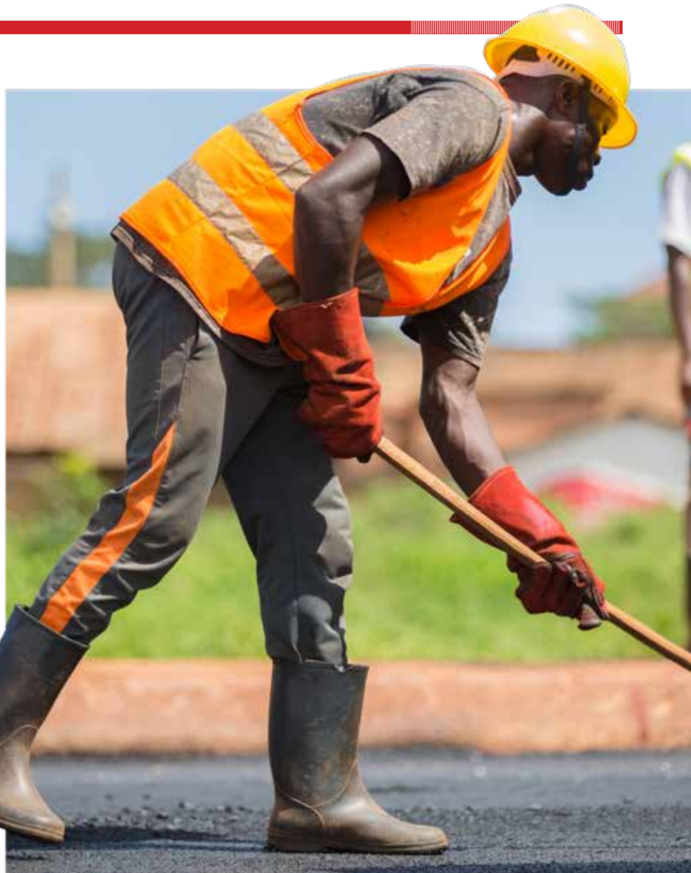
Ongoing road construction works by Abubaker Technical Services & General Supplies Ltd.
