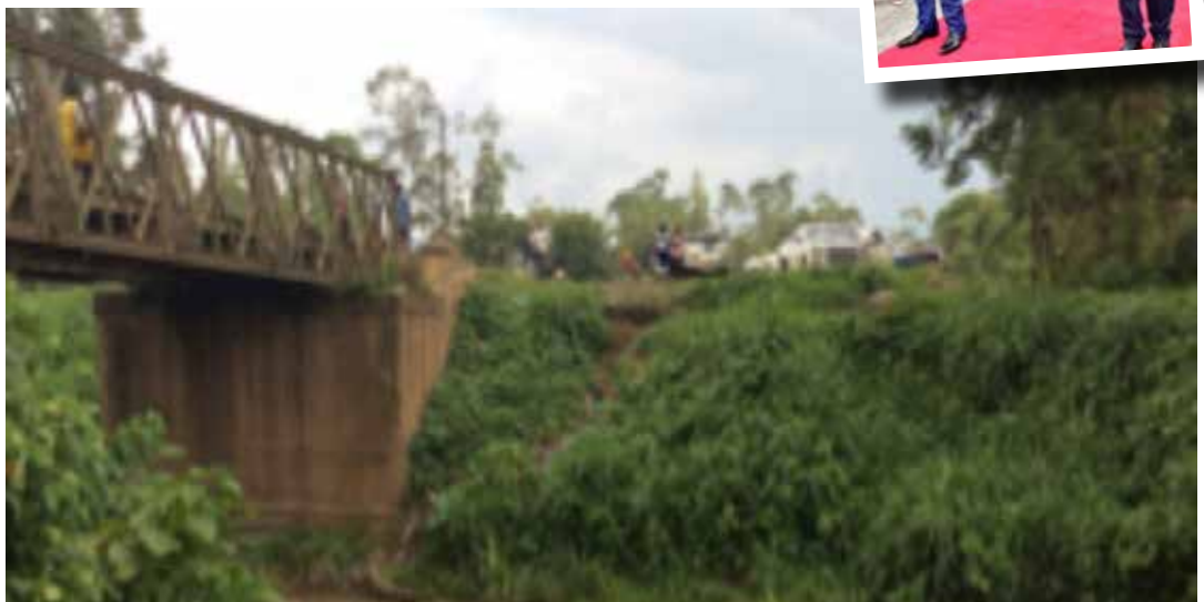
RIGHT: Mpondwe Bridge before construction
