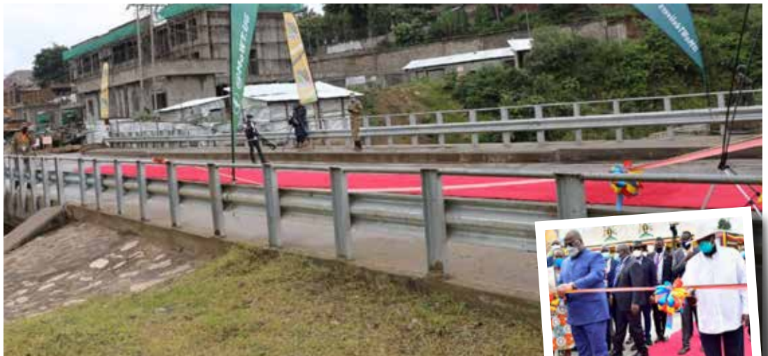
RIGHT: Mpondwe Bridge at Commissioning after completion of construction works
