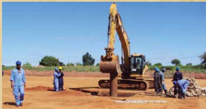
Constructing the cellar Box -To receive the Oil Drill Rig
