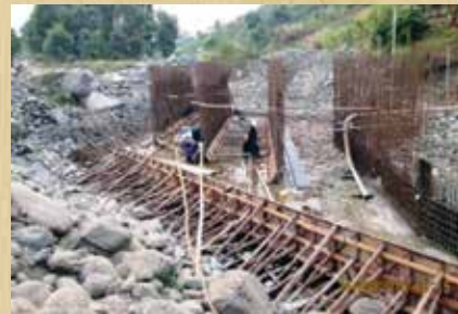
Construction of a Reinforced Bridge -Maliba Bridge at Kasese
