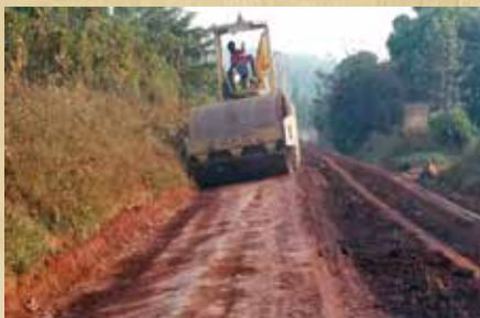
Term Maintenance of Misindye-Namaliri Road ( 3 year Contract)
